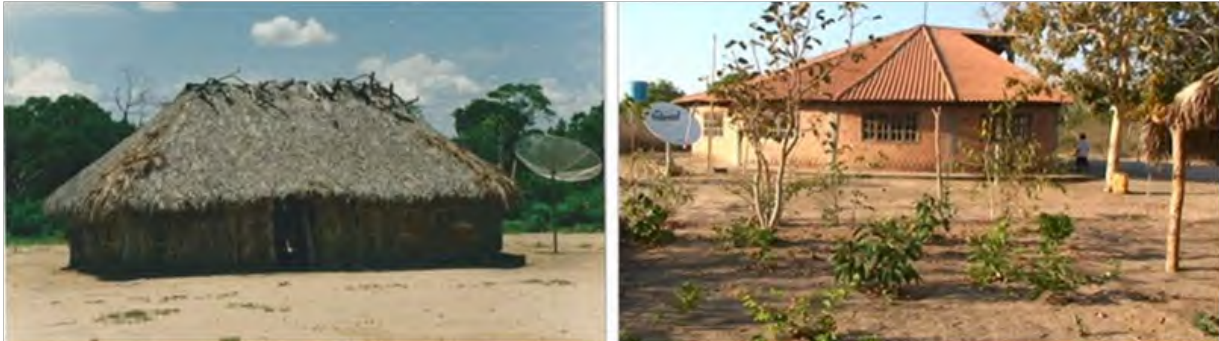
Figure 3 – Wede'rã's Etenhiritipá School – former and current buildings.
